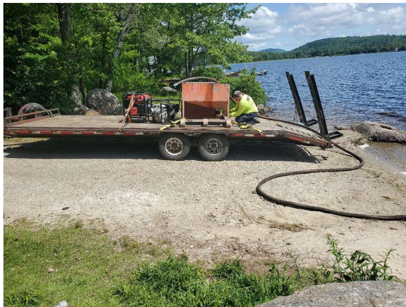
Photo 4 – M&K pump onsite being prepared for final placement
