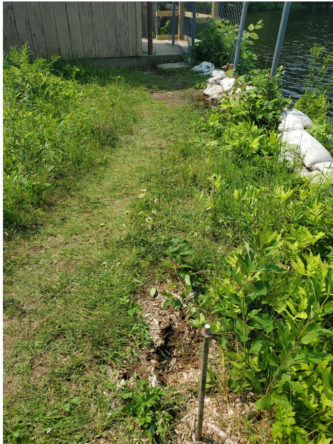
Photo 14 – Sandbags placed to the left of the gatehouse by M&K to prevent overtopping during high water event July 10, 11 and 12.
