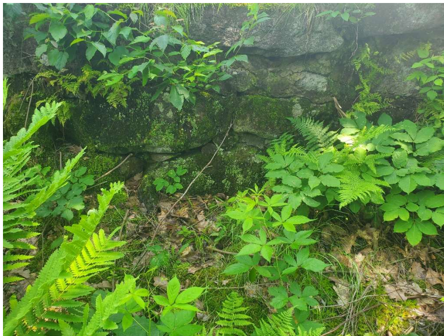
Photo 8 – No observed seepage at downstream toe of dam during high water event July 5, 2023
