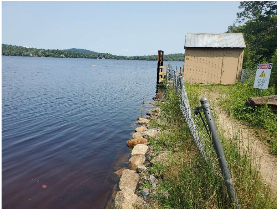
Photo 12 – High water July 12, 2023, water level has reached the low area to the right of the gatehouse
