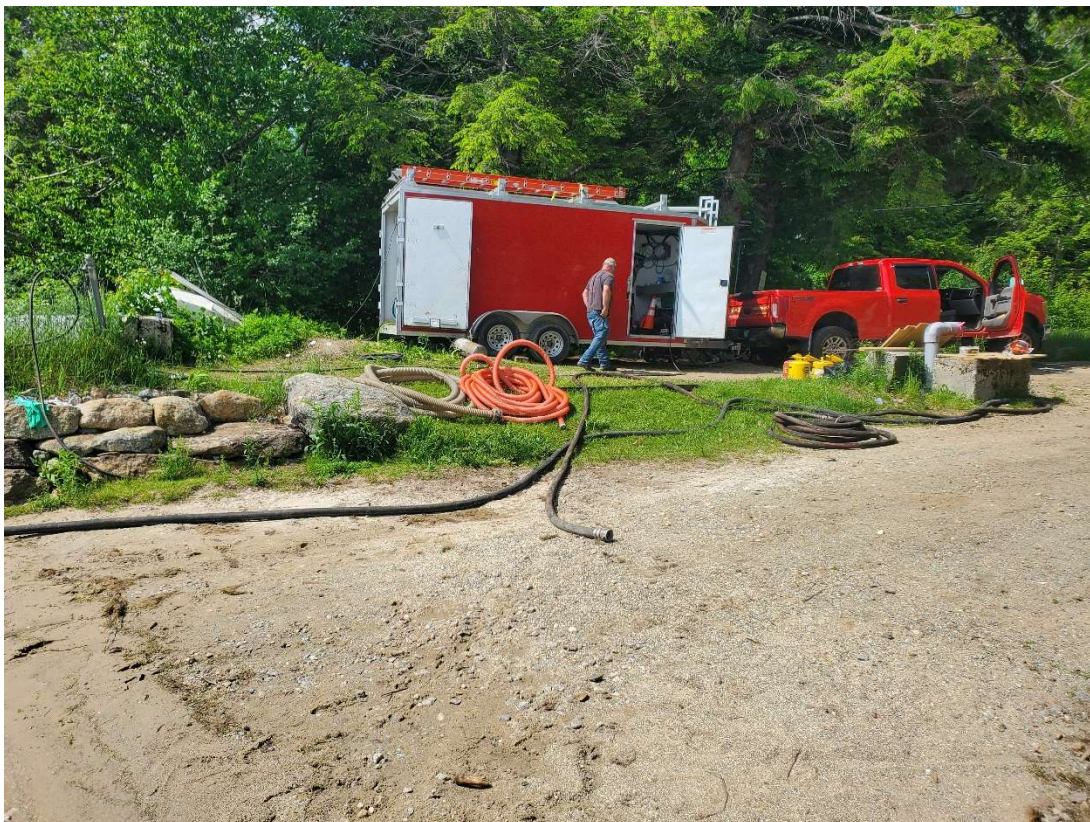
Photo 2 – M&K setting up dive crew control trailer June 21, 2023
