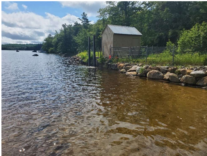
Photo 1 – M&K Divers onsite June 21, 2023 completing additional concrete work at LLO
