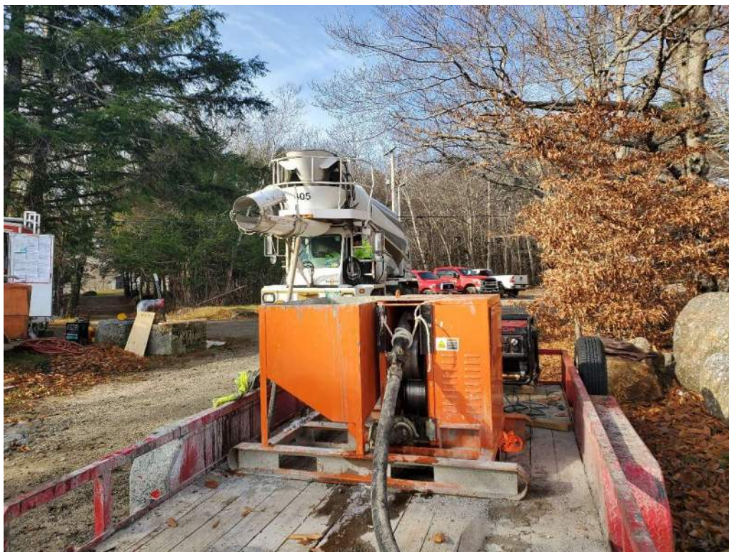
Photo 4 – Carroll Concrete Truck #405 onsite for November 11 placement
