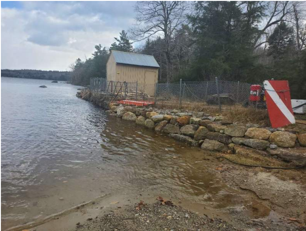
Photo 10 – M&K Onsite installing gate rails
