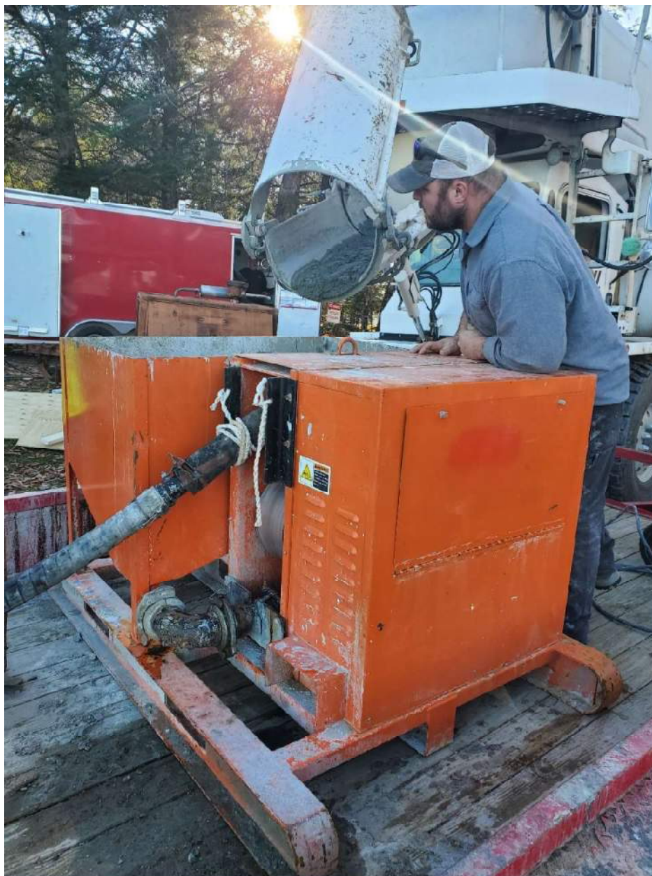
Photo 3 – M&K observing mix condition from Carroll Concrete truck # 405 November 3
