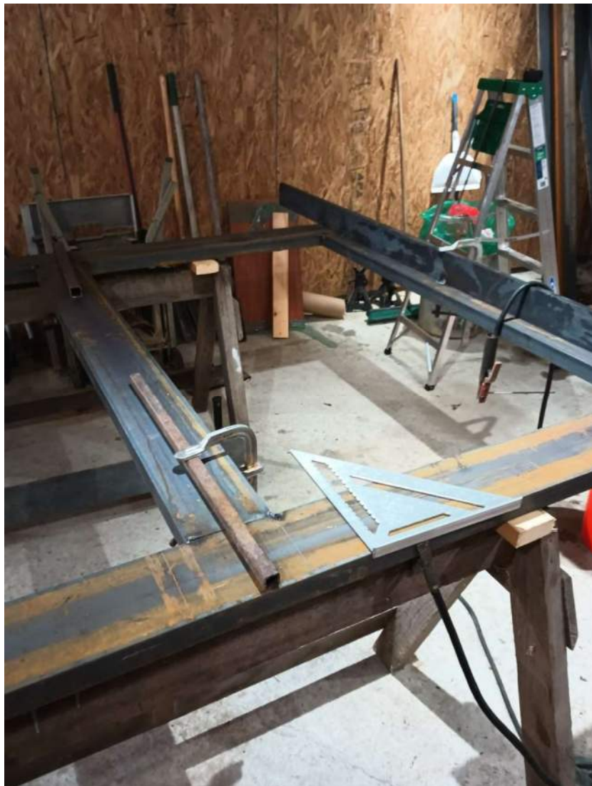
Photo 6 – Gate Rail Fabrication in process
