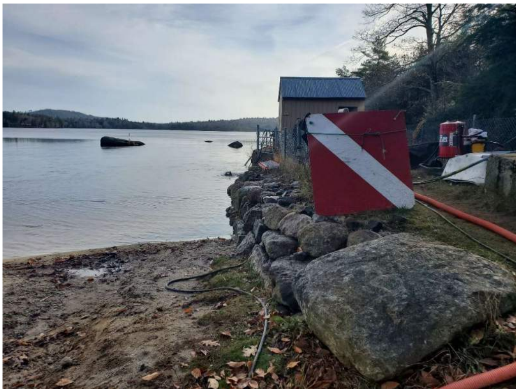
Photo 5 – Dive safety signage at November 11 concrete pour
