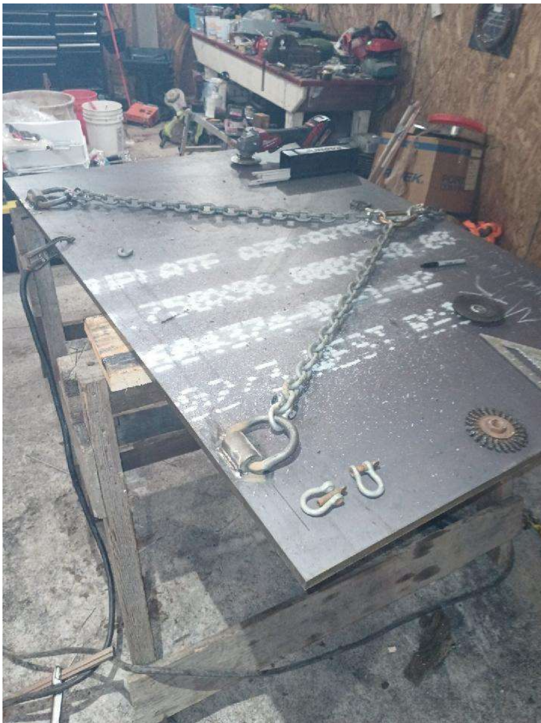
Photo 9 – Gate assembly in fabrication
