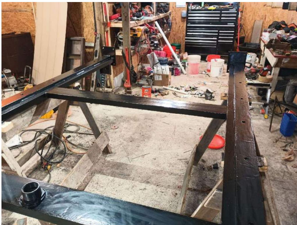
Photo 7 – Gate rail assembly painted
