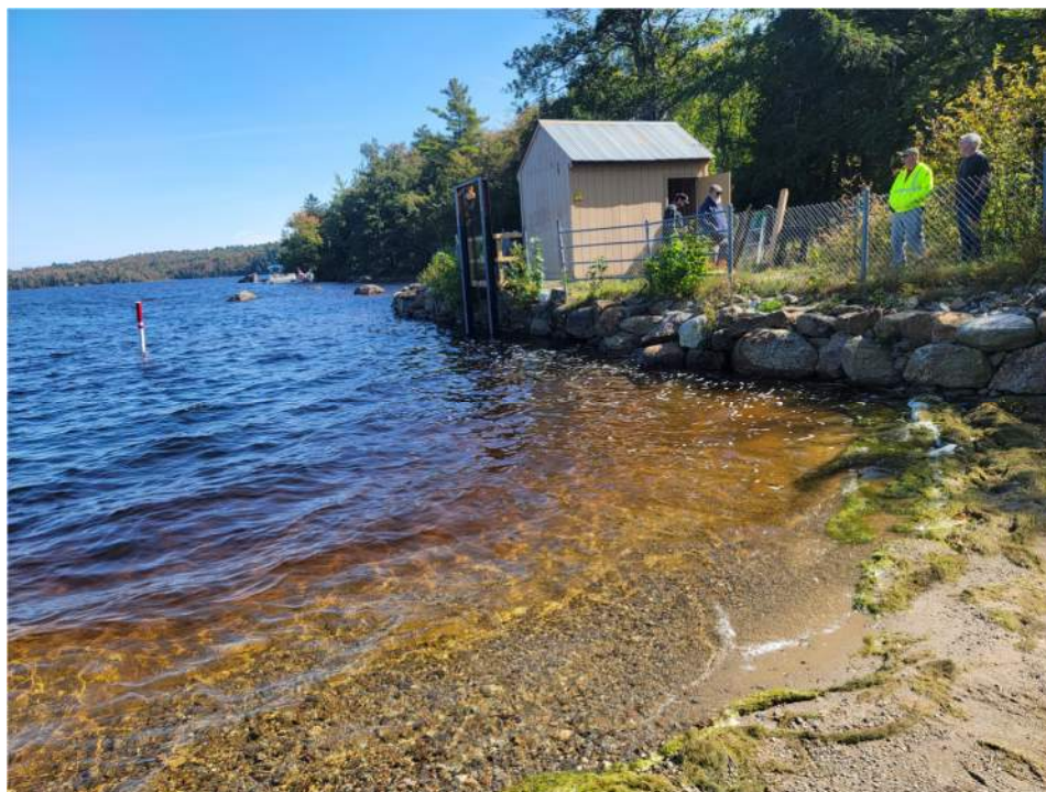
Photo 10 – Ashuelot Pond Dam – upstream face of dam
