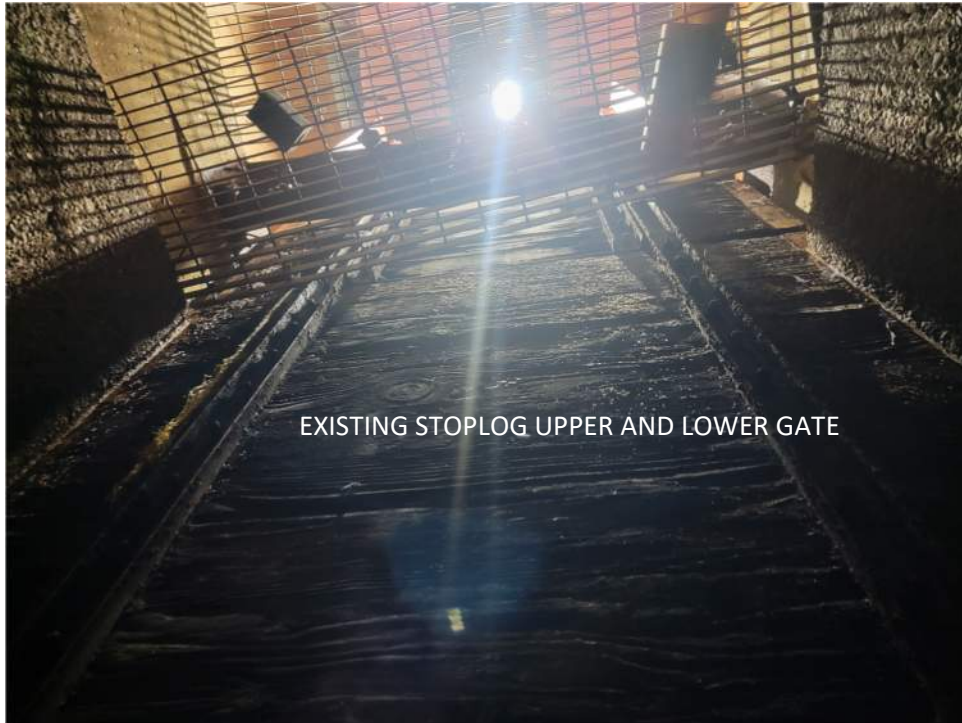
Photo 7 – Ashuelot Pond Dam Gate House – downstream face of existing gate
